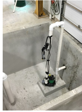
Pump and Floats Assembly
